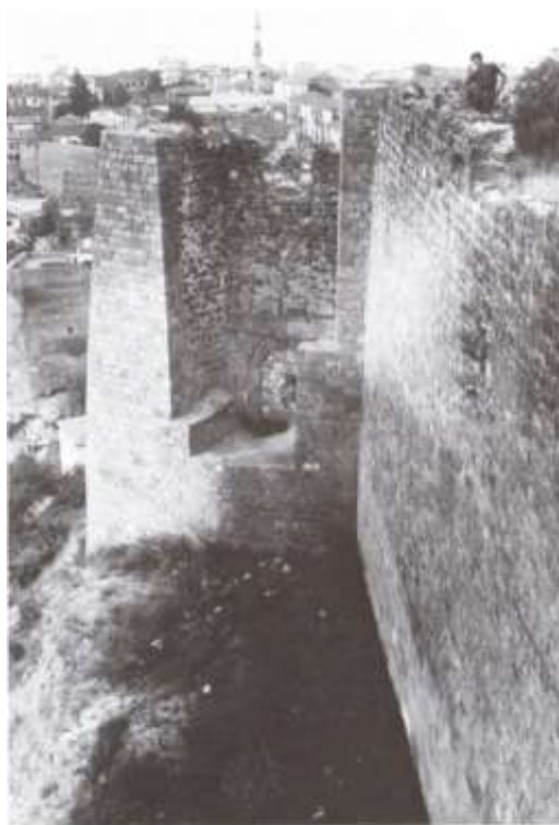
148a. Exedra (Feature 32), mostly refaced, Blocked Door from South
